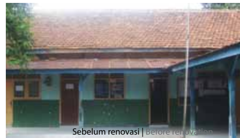
Sebelum renovasi | before renovation
