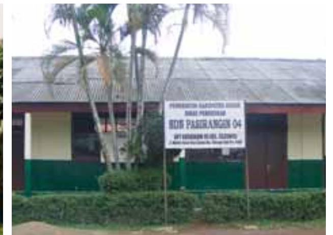
Sesudah Bangunan Direnovasi After Renovation
